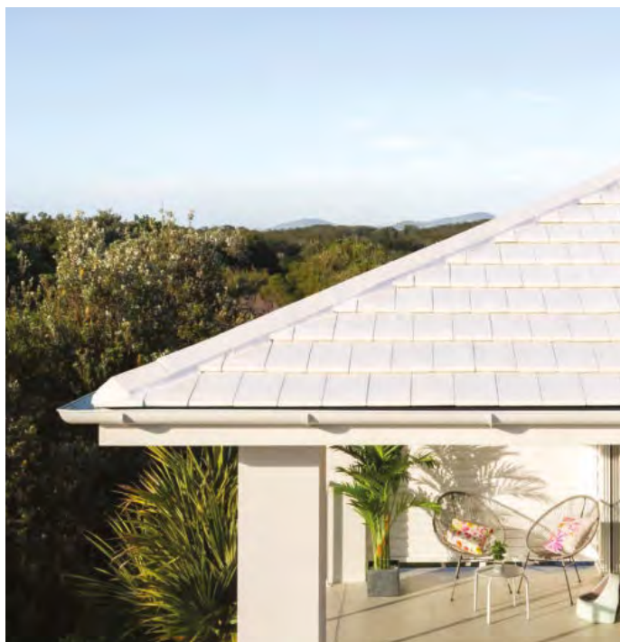
Use of low solar absorption rate materials improves the thermal performance the house
