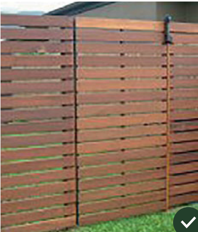
Stained and dressed horizontal timber slat fence and gate
