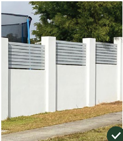
Rendered masonry with horizontal infill panels
