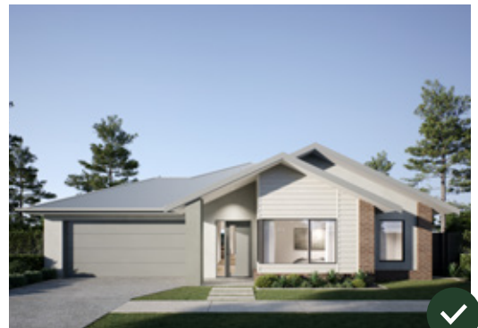
Shaded windows and openings (solar gain protection)
