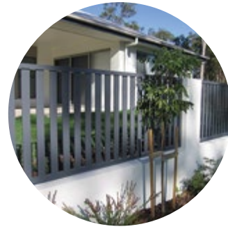
Masonry Front Fence Infill Front Fence
