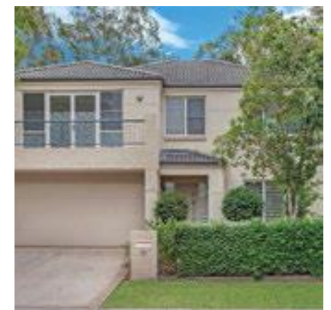
Front garden with well-maintained hedge, strong boundary planting, tree and planting to entry portico.
