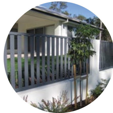
Masonry Front Fence Infill Front Fence
