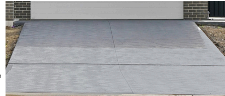
Concrete broom finish (Up to 50 sqm)
