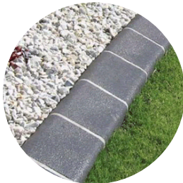
6. FLUSH CONCRETE EDGING
