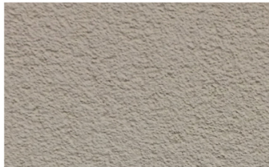
CLADDING* Dulux Pipe Clay
