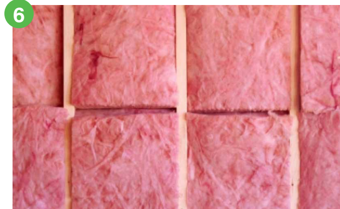
6 Ceiling and Wall Insulation
