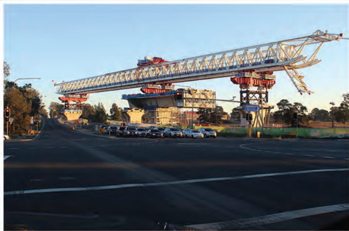
North West Rail Link in construction
