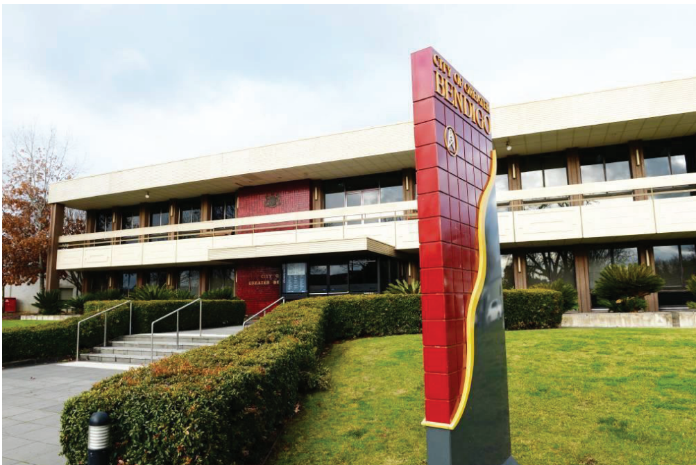
The new Gov Hub will replace the City of Greater Bendigo's main office on Lyttleton Terrace.
