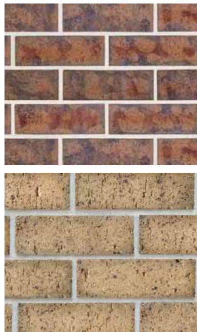
Unaccepted colour variation brick example
