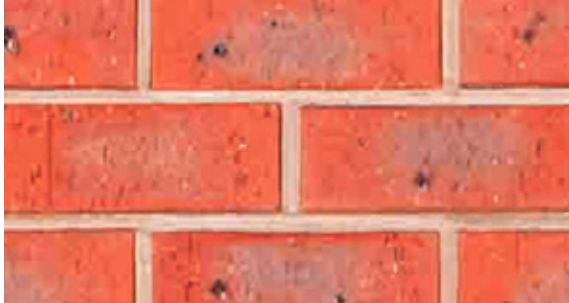
BRICKWORK SELKIRK Copperstone Natural rolled mortar
